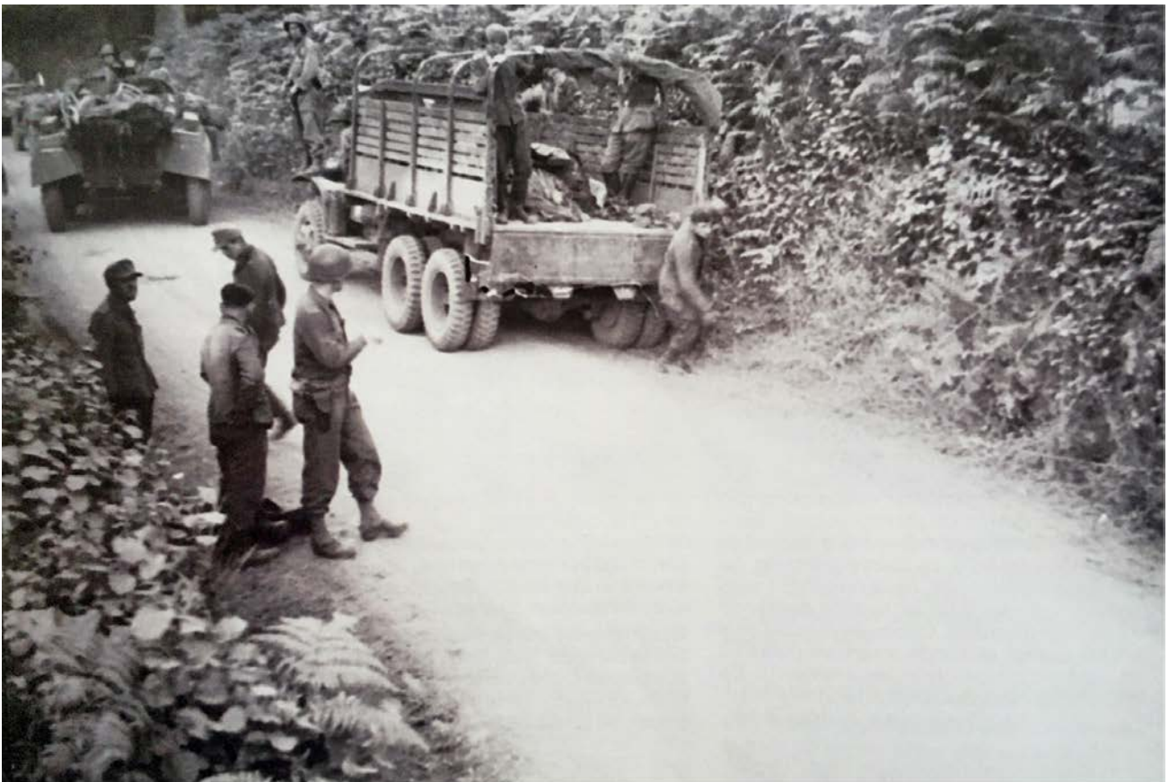
Fig (116) German prisoners collecting dead bodies along the D610 road after the July actions. (USNA)
